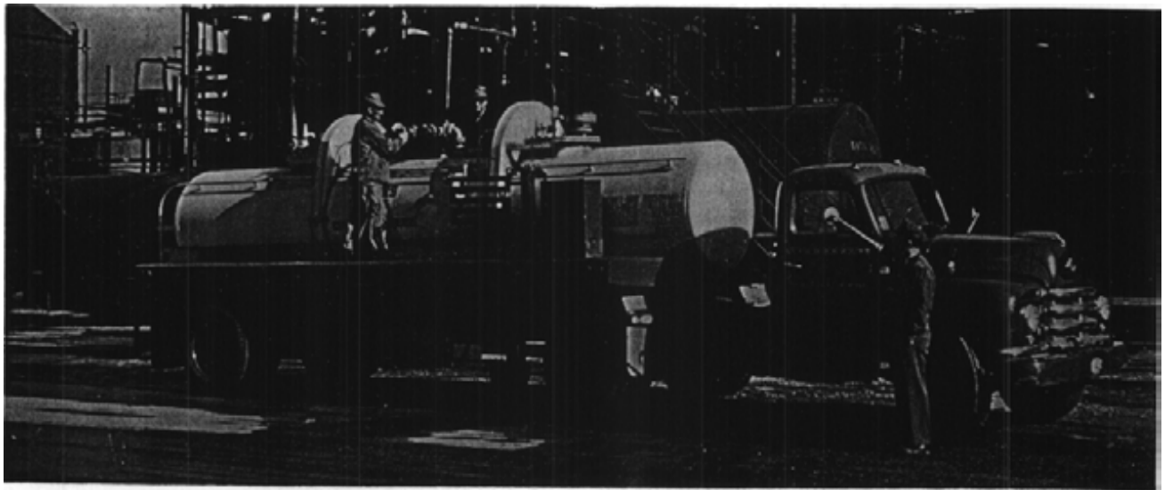
FIG. 17-One of the large companies transports bulk quantities of benzyl chloride in this 2,135-gallon capacity, two-section tank truck. Tanks are constructed from solid Nickel to protect the purity-sensitive chemical from contamination by corrosive attack.
